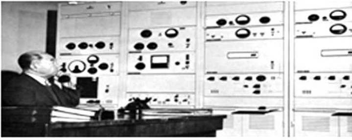
Central control panel at Radio Kabul transmitter in the 1950s.
